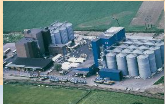
Silo Complex, Svenska Foder, Sweden
