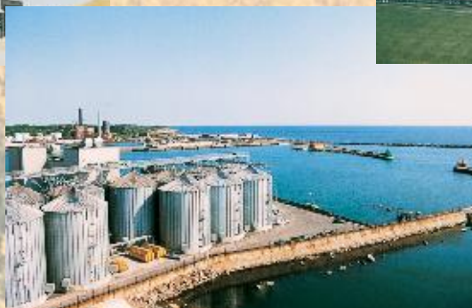
Silo Complex, BAF, port of Rønne, Denmark
