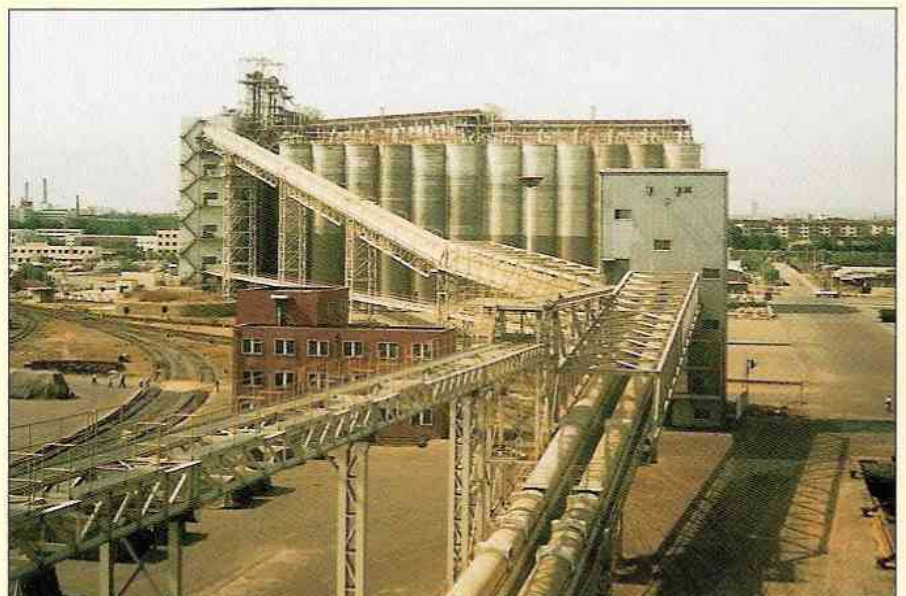
Mitsubishi Heavy Industries, Qingdao, China. Port terminal for import / export of wheat, maize and others. Capacity 660 tph.
